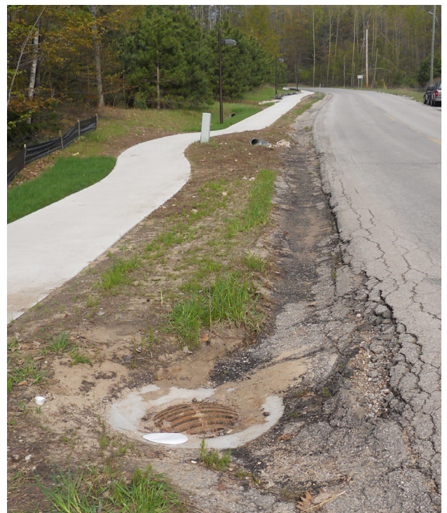
Current stormwater runoff system to Belanger Creek.
