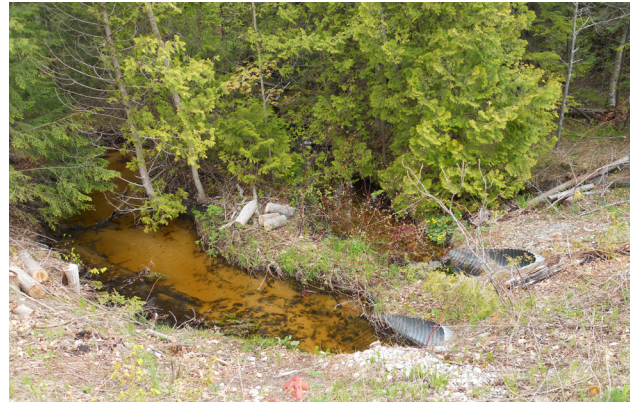
Current Belanger Creek/McKeese Road double culvert road crossing.
