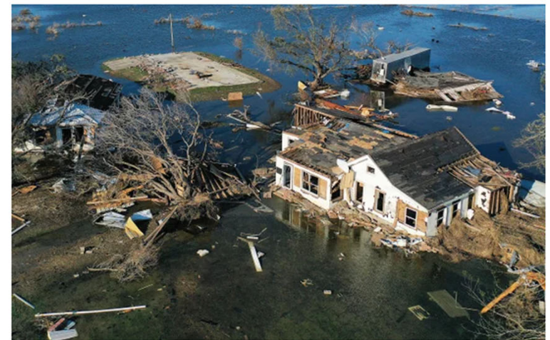
An aerial view of flood waters from Hurricane Delta surrounding structures destroyed by Hurricane Laura on October 10, 2020 in Creole, Louisiana. Credit: Mario Tama Getty Images
