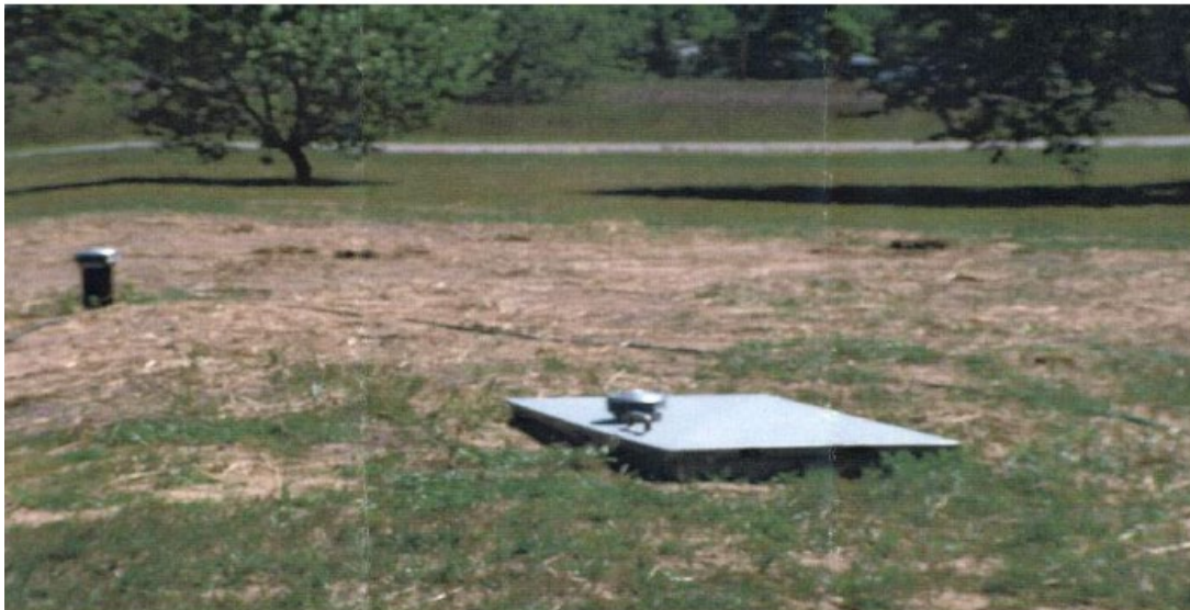
Figure 11. GTB Storm Shelter Entrance in Benzie County
